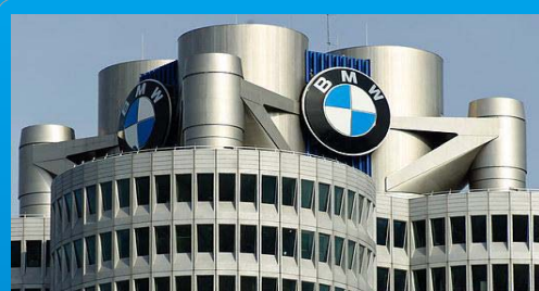
BMW Central Data Center, Munich
