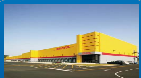
DHL Central Data Center
